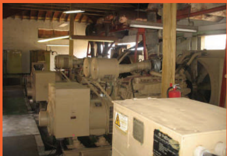
Original Generator Installation
