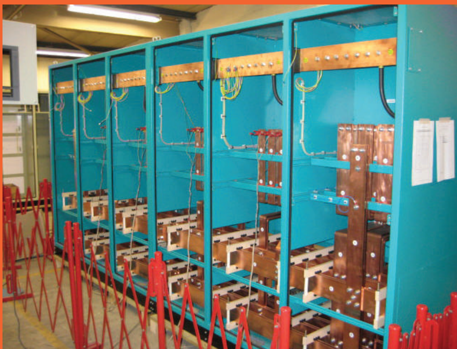
New Control System on test in UK
