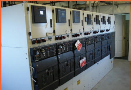
Replacement Gene EVO HV Switchboard
