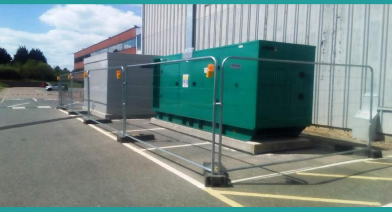
Within this same system the repositioning of an existing 220kVA generator was also required, however due to its condition it was necessary for us to remove it from site and undertake extensive remedial works. The overhaul included our technicians re spraying the canopy and giving it a face lift to its original condition. Once we delivered it back to site we positioned it into the desired location as per the design drawing specification.
