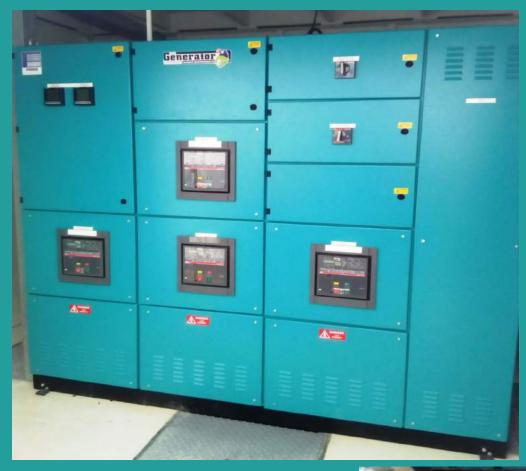
compliant ensuring that when the generators are synchronised with the mains the correct level of protection is available should either supply fail to meet their required standards.
