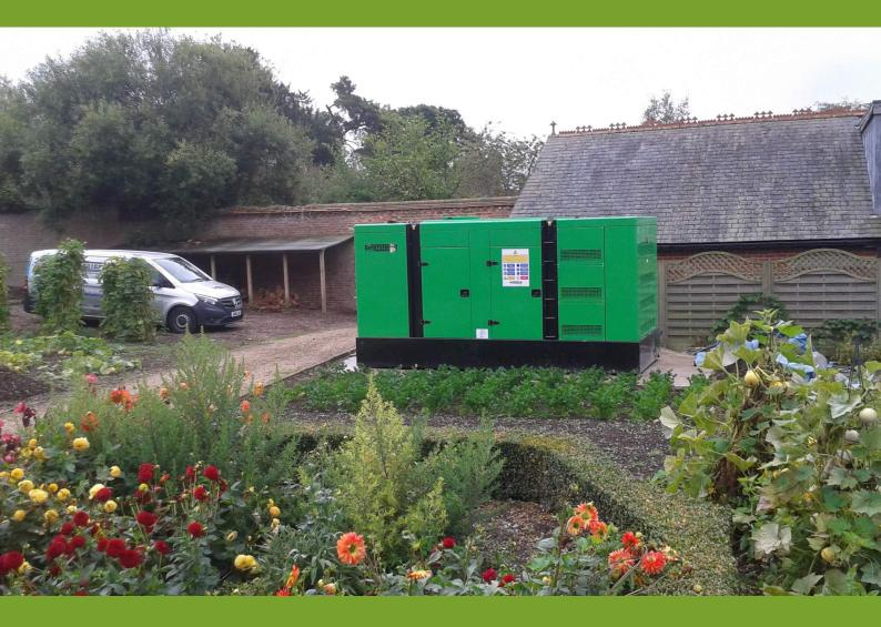
On the agreed date our installation team delivered the 600kVA standby generator to site and manoeuvered it through the archway into the hotel grounds and positioned it onto the hard standing base that had already been constructed. Our engineers then installed the mild steel exhaust system and flexible engine manifold to the generator as per our detailed CAD drawings which had been previously agreed with the client.
