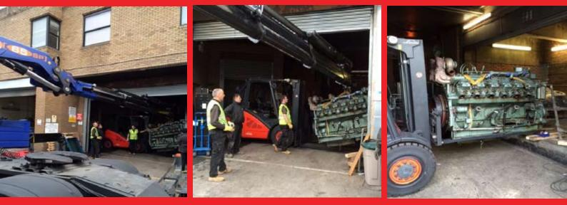
Our Project Manager had planned to remove the existing generators one after the other to ensure that the Hospital's back-up generator power was never below its original capacity.
