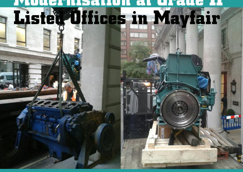
With extensive refurbishments taking place at grade II listed offices in Mayfair, London, The Generator Company were approached for the provision of an upgrade to the property's existing back-up generator power system.
