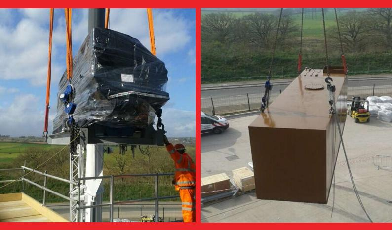
Once it was skated into the correct place the 40,000ltr bulk tank was the next significant piece of equipment to be craned into position followed by the radiator, day tank, exhaust system and attenuation.
