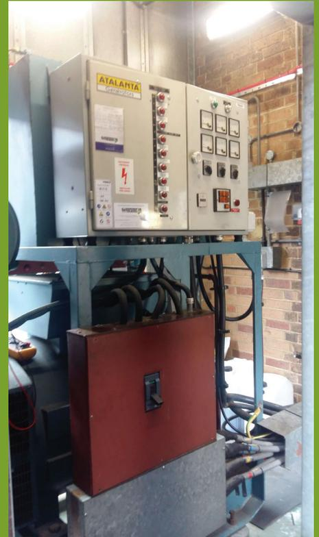
Following a site survey of the existing panels, carried out by our project manager, to assess site conditions and any site constraints, a quote was issued to the client detailing the proposed design, full scope of works and schedule of installation for the upgrade project. The proposed generator control panel will incorporate a Deep Sea Electronics control module and will be designed to allow control as required by the seven existing site changeover panels.
