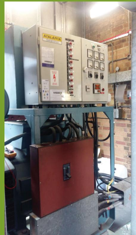
Following a site survey of the existing panels, carried out by our project manager, to assess site conditions and any site constraints, a quote was issued to the client detailing the proposed design, full scope of works and schedule of installation for the upgrade project. The proposed generator control panel will incorporate a Deep Sea Electronics control module and will be designed to allow control as required by the seven existing site changeover panels.
