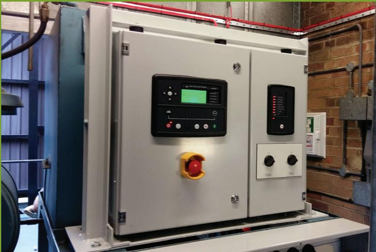
On the specified delivery day, one day prior to installation, all panels were delivered to site. Prior to installation, the generator was isolated and all ATS panels identified and isolated and subsequently disconnected and removed. A new control panel stand needed to be fitted due to the original being part being mounted to the side of the fuel tank.
