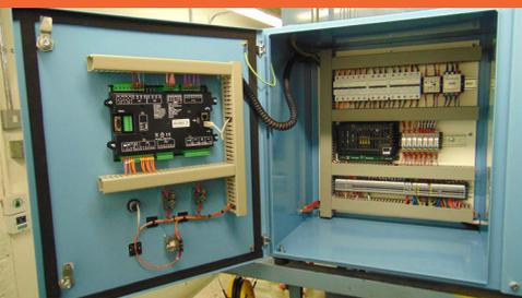
Following completion of the new generator control panel, two generator engineers were booked in over a weekend, due to the nature of the business this could not be done during normal working hours, to remove the original Autodiesel Control Panel and replace it with the new DeepSea Control Panel.
