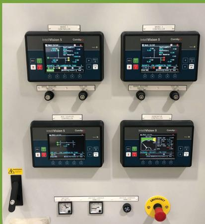
A black building test was carried out, resulting in the electrical power to the entire building being shut off to simulate a total power failure allowing us to test the functionality of the generator and ancillary equipment, both of which was successful.
