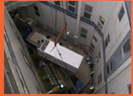
Attenuator craned onto plinth
