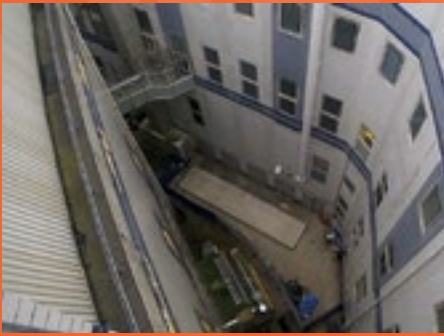
Prepared concrete plinth in courtyard
