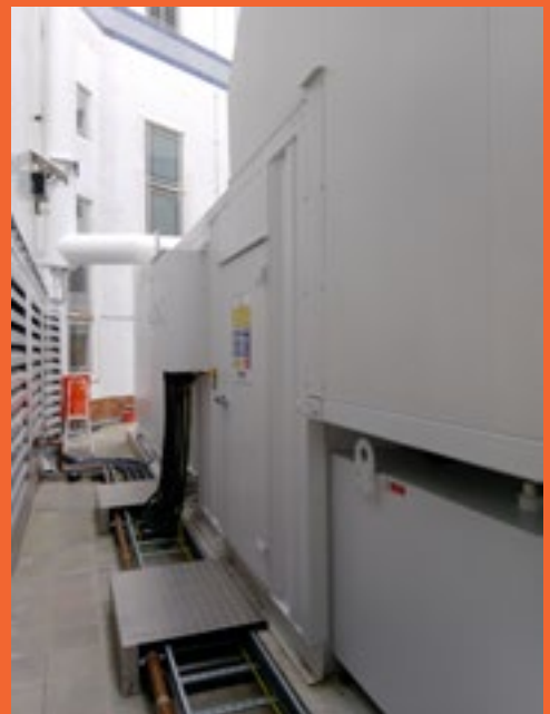
Final installation of all equipment
