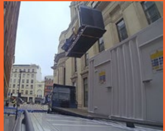
First crane lift adjacent to the building
