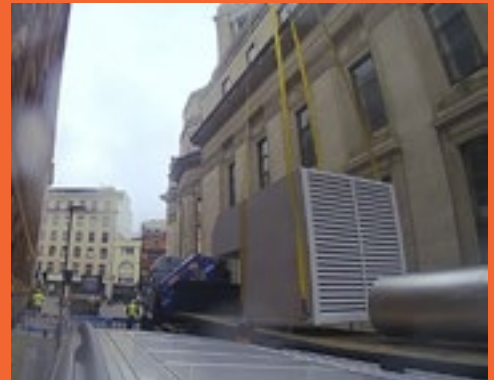
Second crane lift
