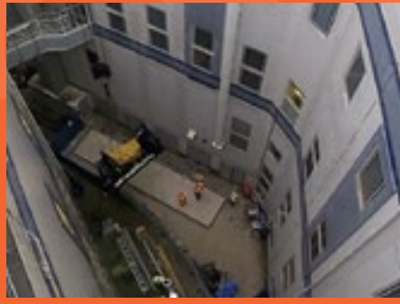
Generator craned onto plinth
