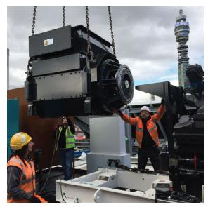
The installation of M&E works was completed over 4 months with numerous co-ordination and design meetings required to finalise the routes for the fuel system pipework and control cables for the master control panels between the generator located at roof level and bulk fuel tank and master control panels at basement level 2.
