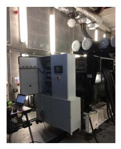
The proposal was modified on request of the end-client due to changing of suppliers during the tender process, with the generator resized to 1 off 2500kVA with an oversized alternator to meet the revised load profile, thus reducing the footprint area of the generator.
